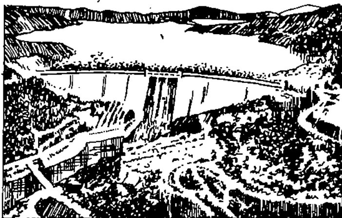
Fig. 8.2 : A reservoir formed behind Shastri Lake showing two possible means of releasing water from impoundments
